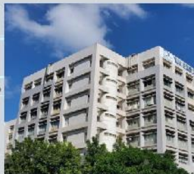
New Taipei City Headquarters Office Factory 1
